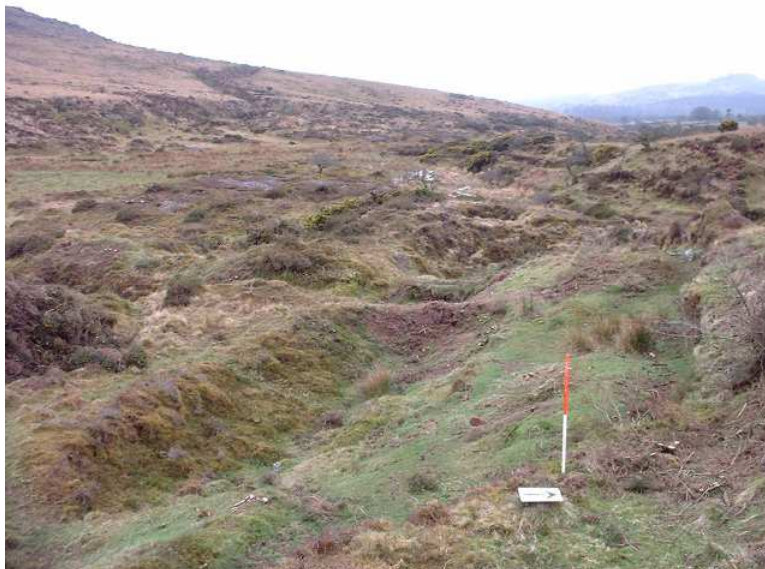
Fig 19 Plym Consols Mine after clearance. Processing area and wheelpit in centre of photograph, shaft and bob pit beyond
