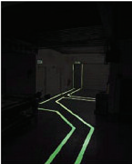
Figure 63: A 'way-guidance' system
