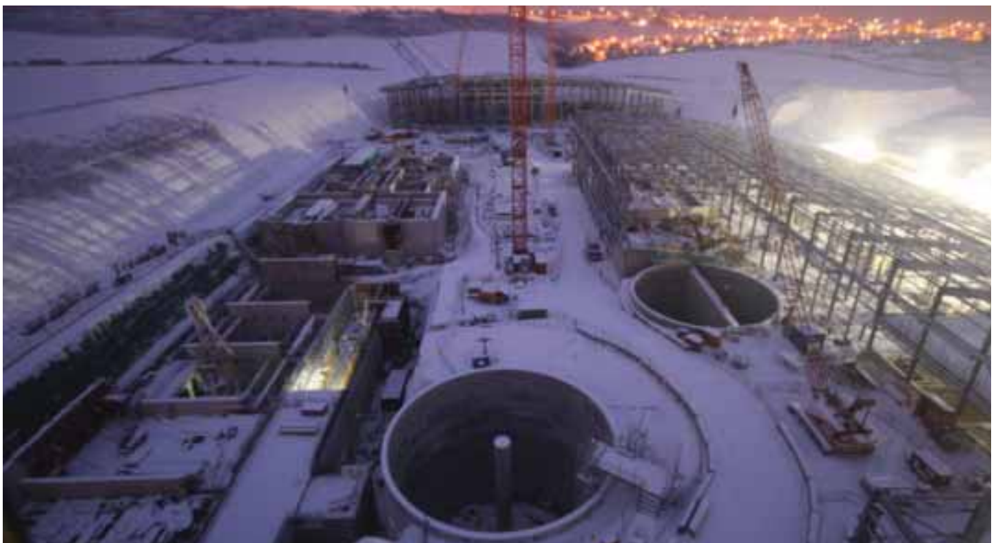
Figure 2: Brighton and Hove treatment scheme in construction – December 2010
