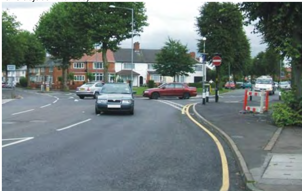
Photo 3.16: Cotterills Lane/Alum Rock Road realignment (old kerb line runs adjacent to tree)
