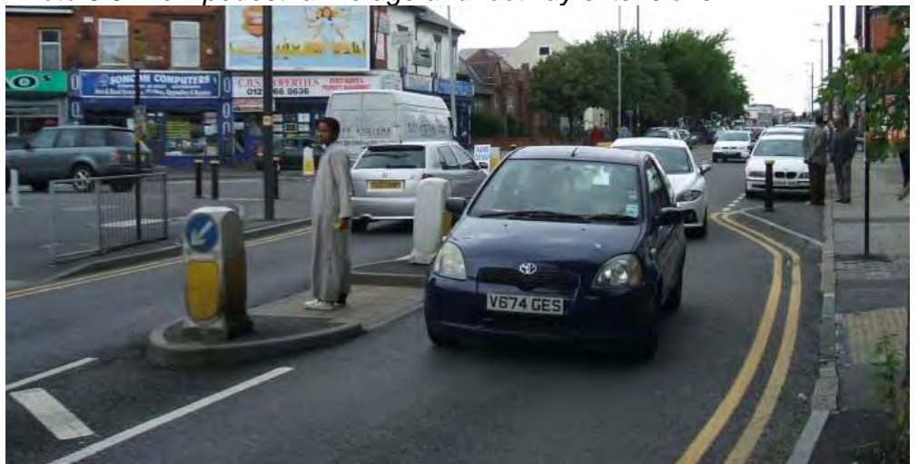
Photo 3.8: New pedestrian refuge and footway extensions
