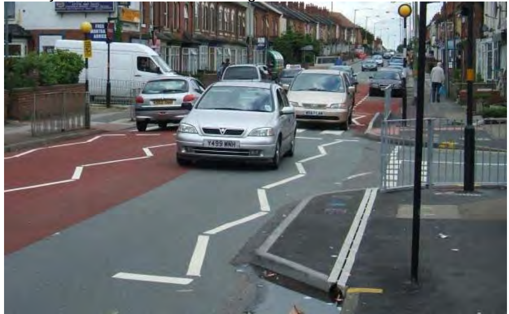
Photo 3.10: Green Lane /Third Avenue – carriageway narrowing and footway extensions at zebra crossing
