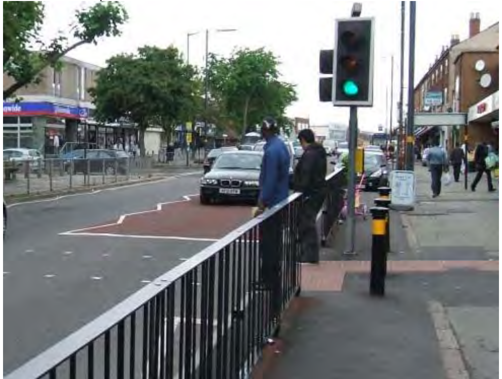
Photo 3.7: New pedestrian crossing facility (note old kerb line to the right of the bollards)
