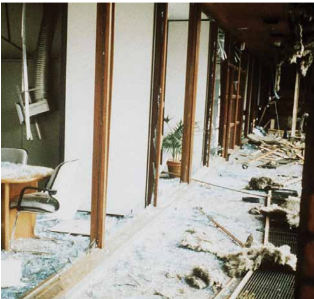
The effect of a blast on laminated glass - top picture, compared to toughened glass - bottom picture.
