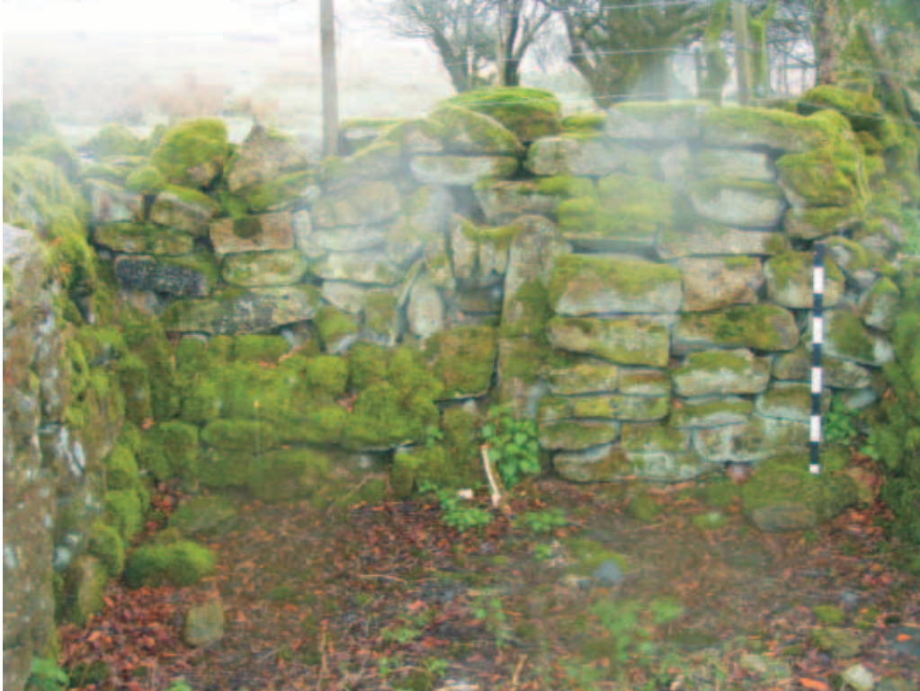
Plate 29; Inside elevation of south wall of calf shed, 2006, scale 1m
