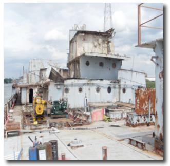
Dismantling forward structure removed up to the funnel
