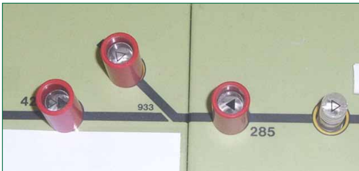
Figure 12: Typical reminder devices (red tubes around the press button) used on a control panel. A press button without a reminder device is on the right-hand side of the picture
