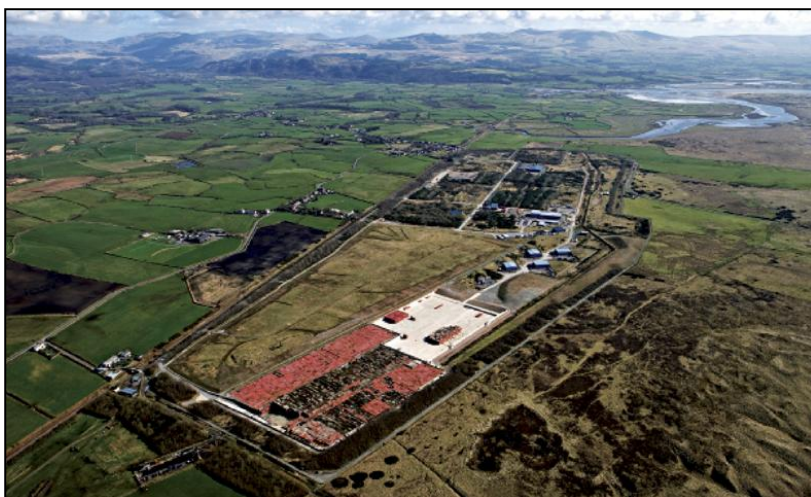
Figure 1: Aerial view of the LLWR viewed from the north-west (courtesy of LLW Repository Ltd)
