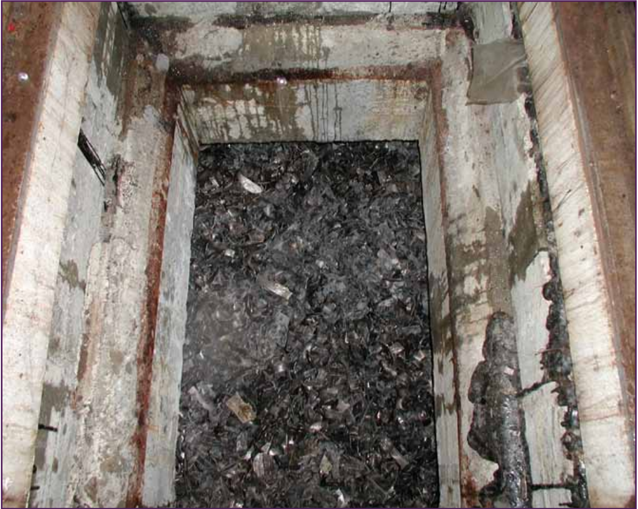
Dissolution can reduce the volumes of FED currently stored in Bradwell's vaults by up to 97%
