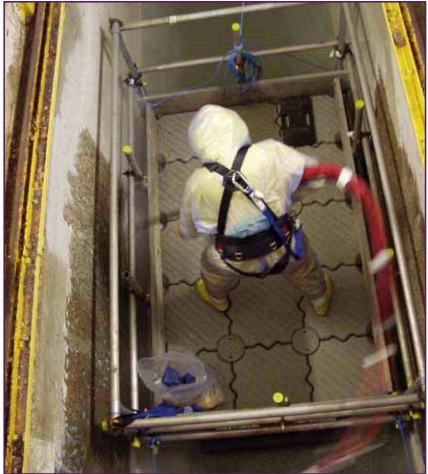
Ultra high-pressure washing of the walls from a floating pontoon
