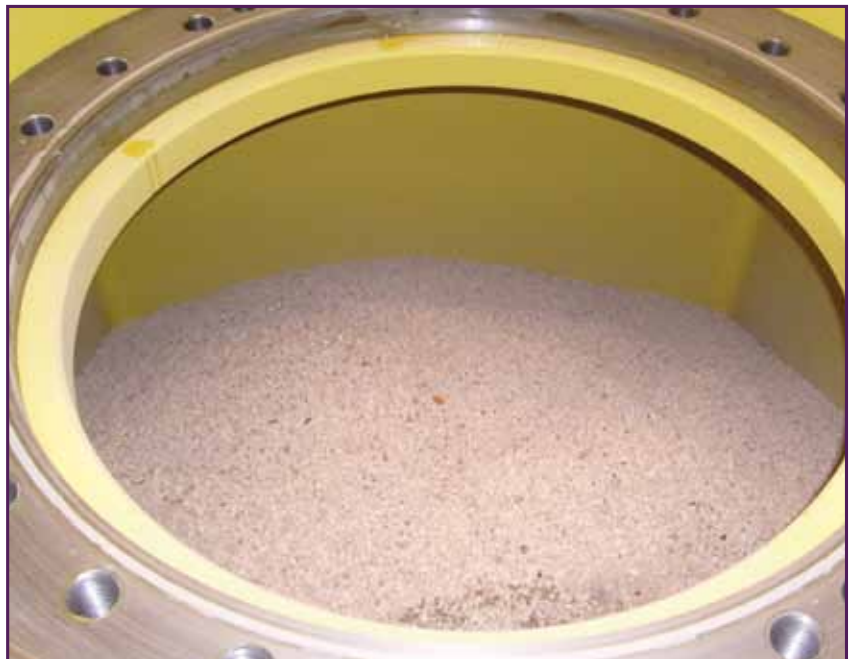
Desiccant, successfully transferred to GNS Yellow Boxes at Bradwell and Wyffa
