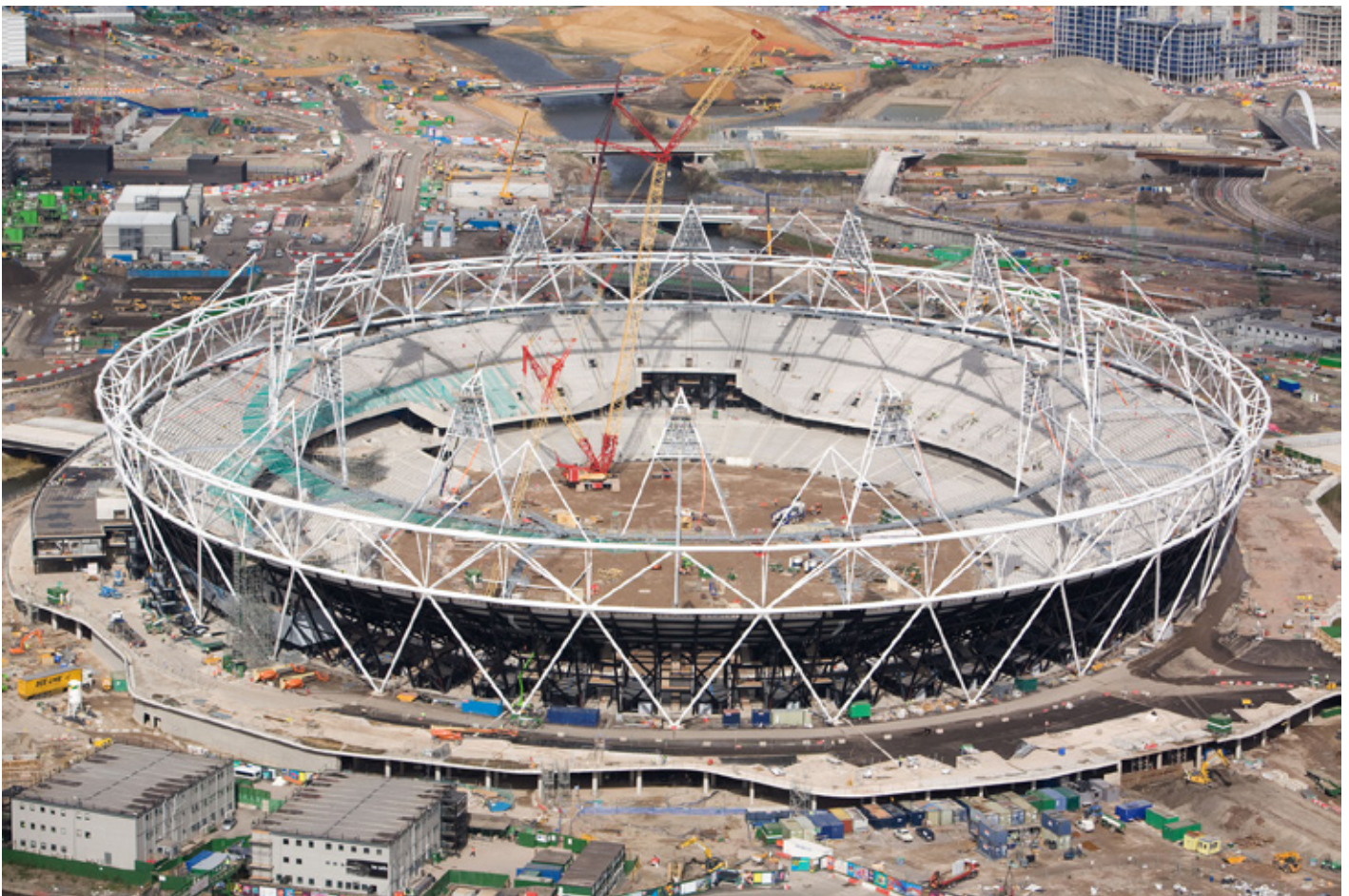
Construction of the Olympic Stadium.
