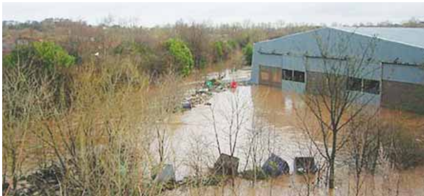
Photograph 1: Flooding through the Willowholme Industrial Estate, Carlisle.
