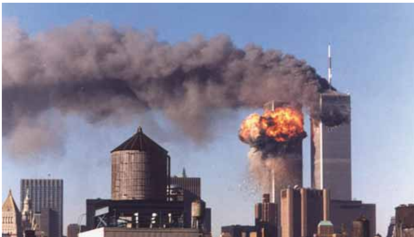
Photograph 1: The impact, fireball and atmospheric plume.
