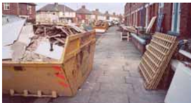
Photograph 2: Skips containing flood damaged materials in a Carlisle street. © Chemical Hazards and Poisons Division.
