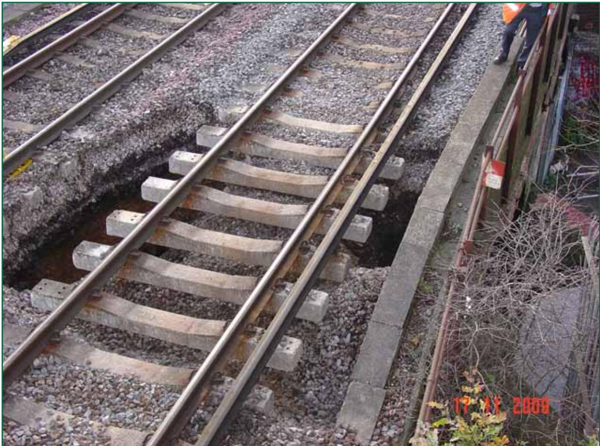
Figure 7: Overview of track showing loss of support to up line
