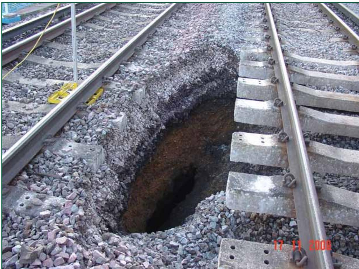
Figure 8: Void to river in six-foot between up and down lines
