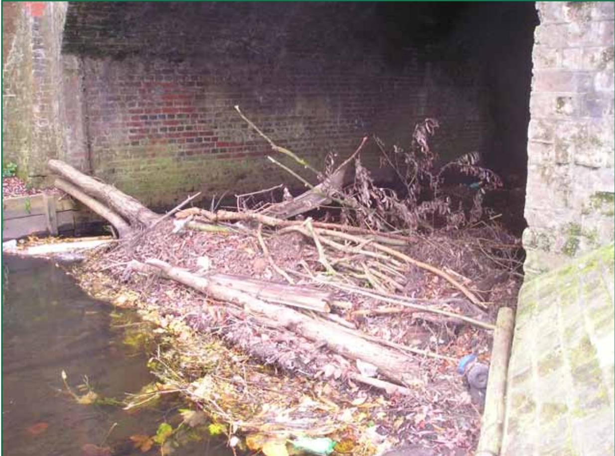
Figure 5: Obstruction across upstream face of bridge 48 on 28 October 2009 (photograph: Environment Agency)
