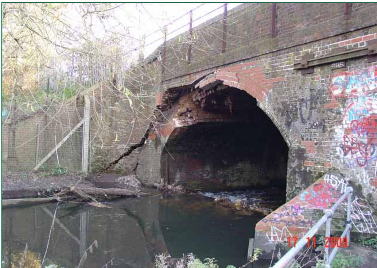
Figure 6: upstream face of bridge 48 following the incident showing failed arch
