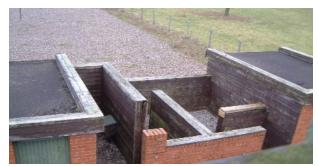
(b) **Tactical Grenade Range**. A tactical grenade range, for use by trained personnel, on a LFTT Area. It may comprise only protection for tactical grenade throwing as set out in Reference B (PAM 21) or temporary or permanent structures with protection as illustrated in Figures 22-2 to 22-6 and set out in Reference B
