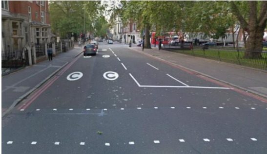
A4200 Eversholt Street (looking south)
