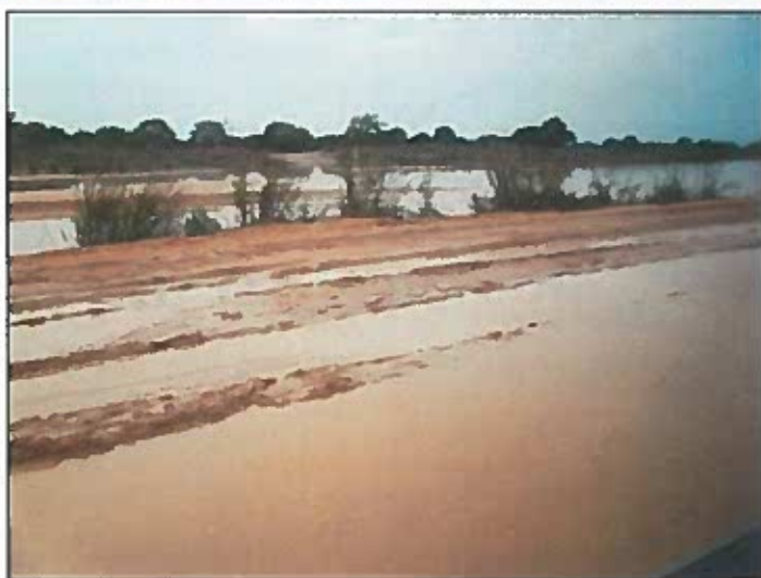
Figure 5-90: Road linking Luanda to Soyo.
