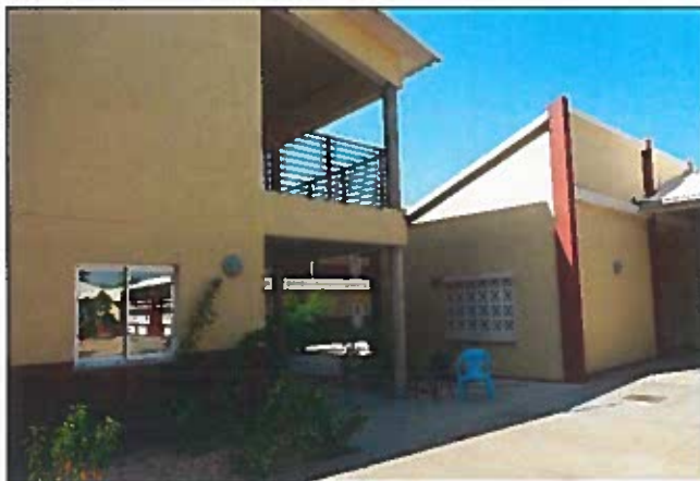
Figure 5-114: Primary School No. 2 Facilities.
