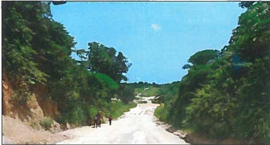
Figure 5-88: Access to rural community.
