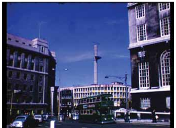
St John's Beacon under construction 1957-58.
