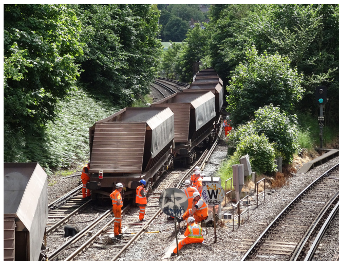
Derailed freight train at Angerstein Junction (10/2016) (courtesy of Network Rail)
