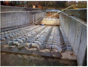
Construction has finished on the major new fish pass at Sprotbrough, River Don. Once opened, the pass will allow fish access to 8 miles of river upstream of Sprotbrough and at least 3.5 miles of the River Dearne. Coarse fish will be able to reach spawning grounds which have, until now, been inaccessible. The project is a partnership between the Environment Agency, the Canal and Rivers Trust and LaFarge.
