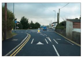
Photo 3.13.4: Traffic calming on approach to mini-roundabout
