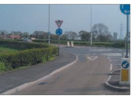
Photo 3.6.1: Example of mini-roundabout within 40 mph speed limit with constrained approach
