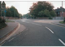
Photo 4.2.9: Mini-roundabout with overrun area
