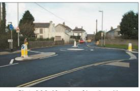
Photo 2.3.2: After view of junction with mini-roundabout
