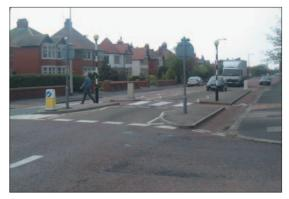
Photo 3.7.3: Mini-roundabout incorporating segregated cycle facilities and zebra crossing
