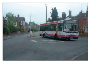
Photo 3.13.1: Bus at mini-roundabout with severe deflection
