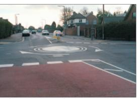
Photo 2.1.3: Non-conforming concentric rings
