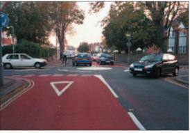
Photo 4.2.10: Mini-roundabout with red anti-skid
