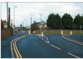
Photo 4.2.4: Deflection through alignment and traffic island
