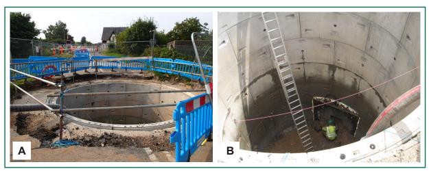
Figure 6: Launch shaft (a) and reception shaft (b) during the works (image courtesy of Morgan Sindall)
