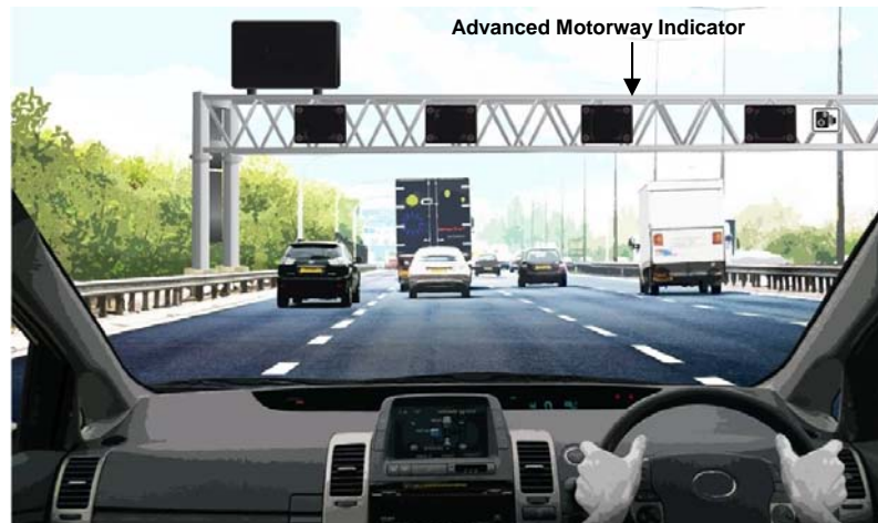
Figure 4A: Illustrative M3MM section operating in normal motorway conditions with blank Advanced Motorway Indicators and blank gantry mounted Variable Message Sign
