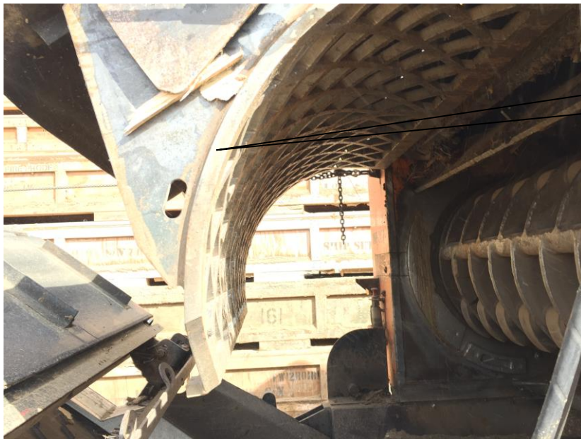
Rubber damping to hammer mill
