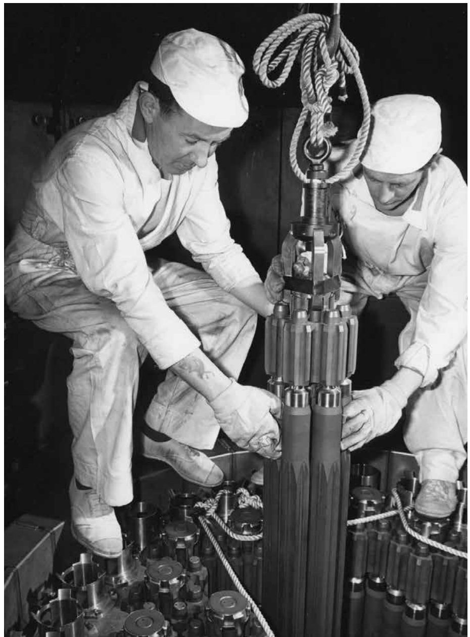
The camera shows a close-up of the control rod guide tubes. Below, fuel being installed during the 1960s.
