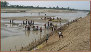
Nepal: barriers to disaster Nepal is prone to natural hazards, of which flooding is both the most common and most damaging. Building flood barriers from local stones, reeds and wood helps communities control the extent to which floods affect their lives.
