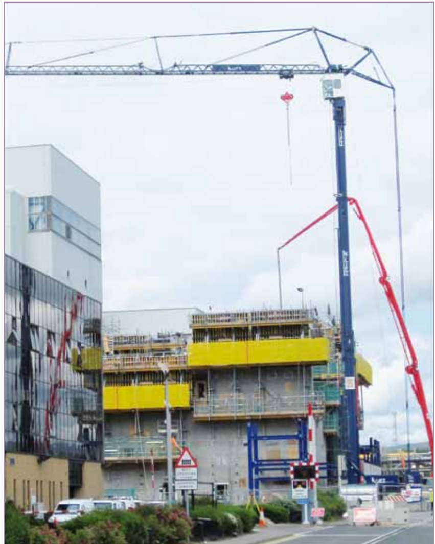
The cranes are designed to fold down when not in use
