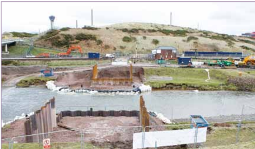
Above: Preparations are made for the temporary bridge
