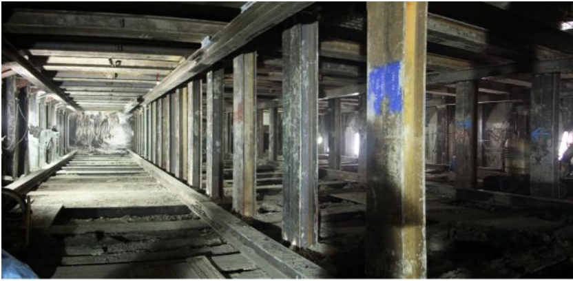
DTL1 Bugis Mining under operational station
