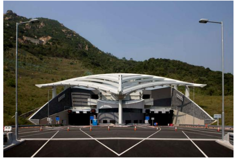
Route 8 Nam Wan Tunnel, Hong Kong
