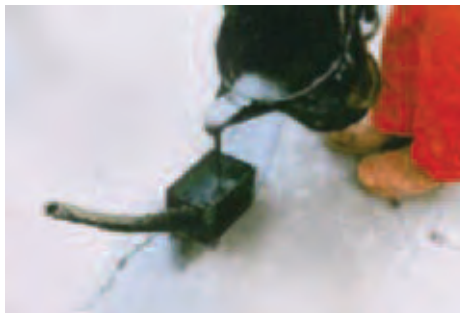
Applying hot overbanding using a screed shoe
