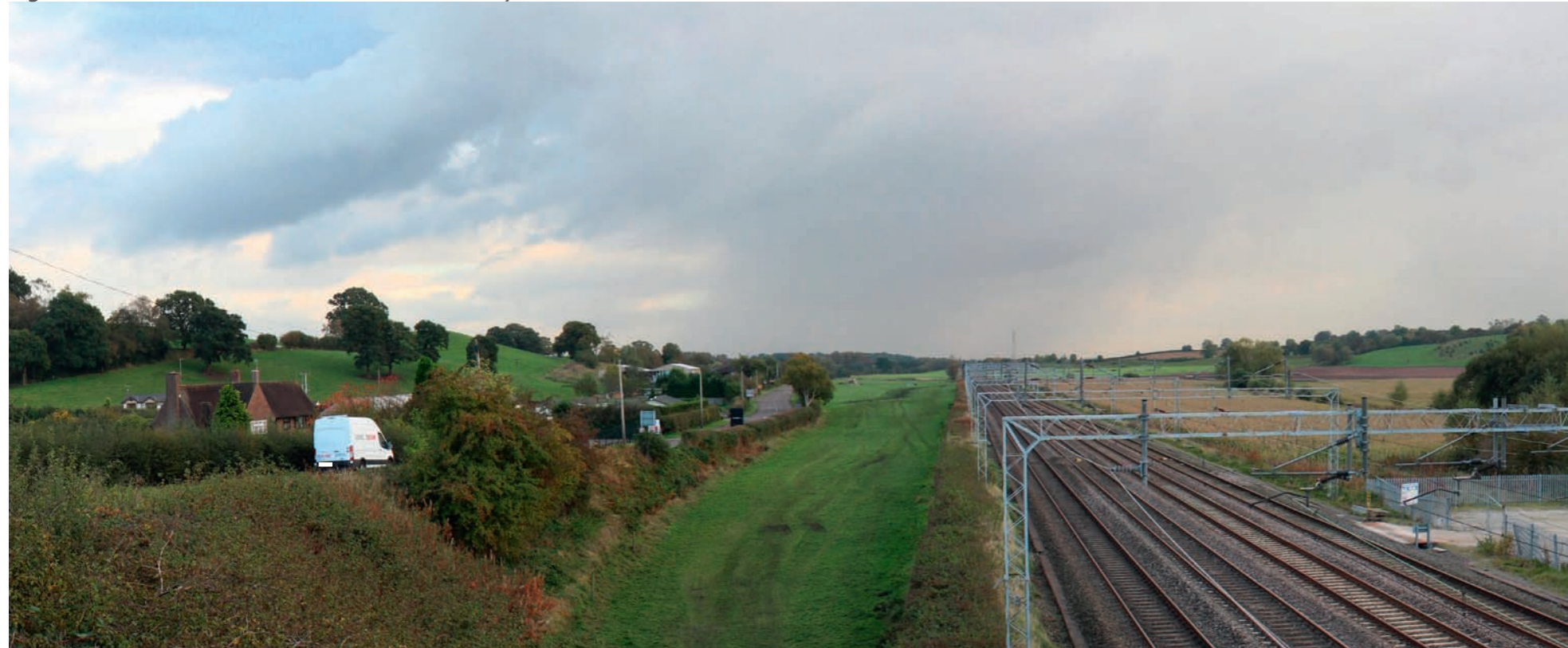
Figure 4: View of WCML within Meece Brook valley
