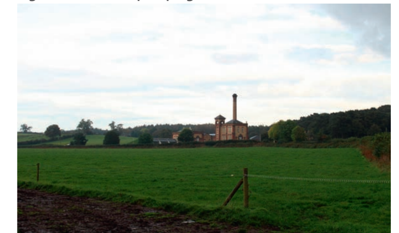
Figure 3: Victorian pumping station
