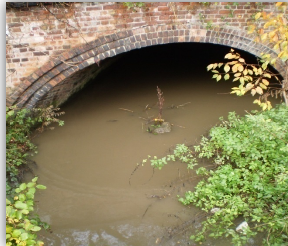
Cudworth Dike, River Dearne, South Yorkshire
