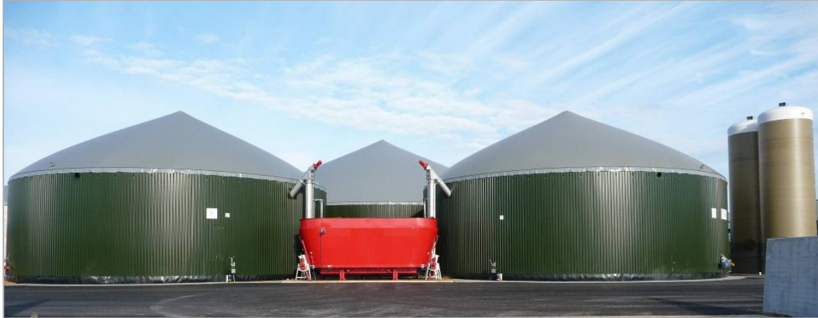
Figure 3:12: Anaerobic Digestion Tanks Showing 2 Primary Digestion Tanks.
