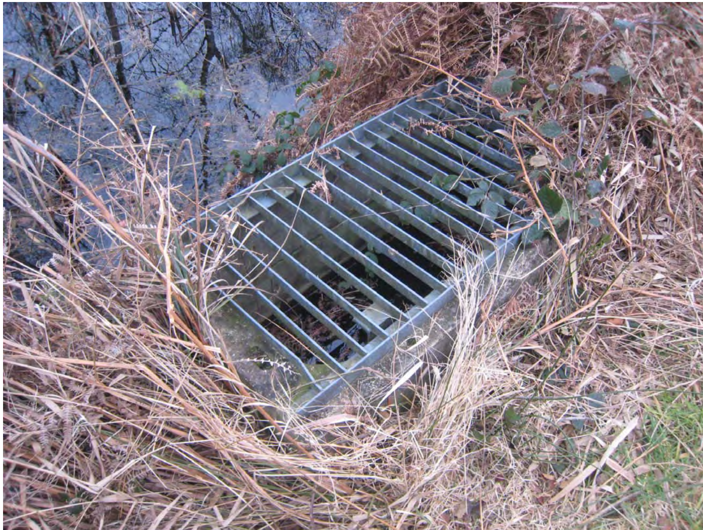
Figure J2 Close-up of the northern sluice showing the wooden boards (27/2/2012)
