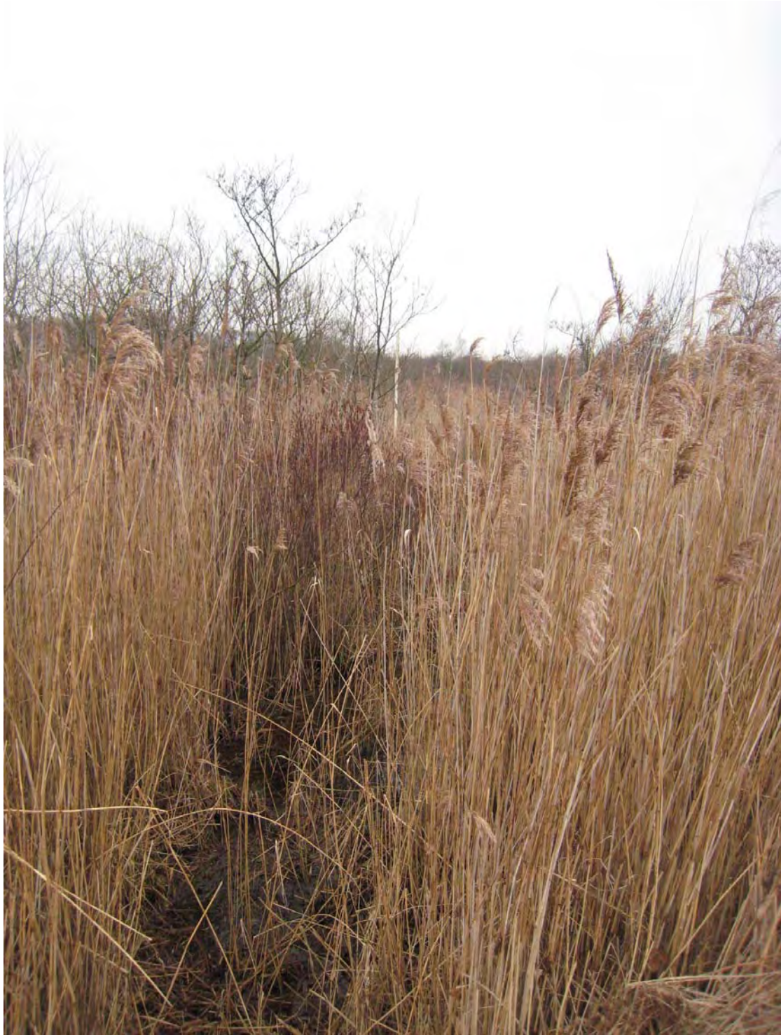
Figure J5 External dyke separating the Commissioners' Rond from the line of dipwells (marked by white posts) in the southern part of Great Fen. The dyke is very overgrown. Gaugeboard NTG3261G2 is located in the same dyke further north, with the dyke being similarly overgrown. Photograph from Commissioners' Rond looking west (27/2/2012)
