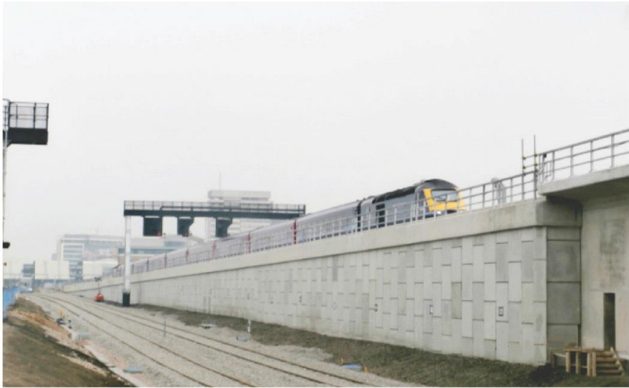
Similar Use of Reinforced Earth Wall
