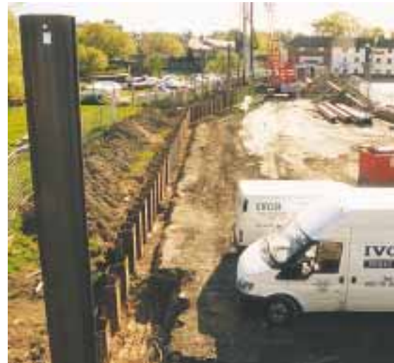
Building the flood defences, Frankwell, April 2002
