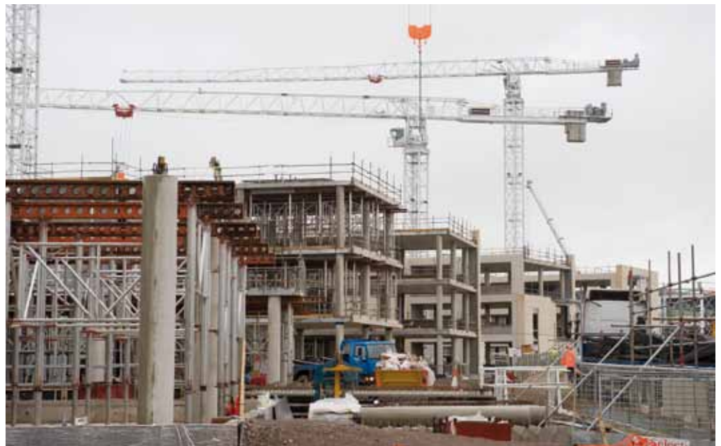
Above: redevelopment continues at pace at Corsham
