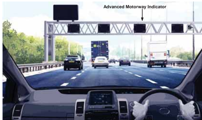
Figure 4A: Illustrative M25MM section operating in normal motorway conditions with blank Advanced Motorway Indicators and blank gantry mounted Variable Message Sign
