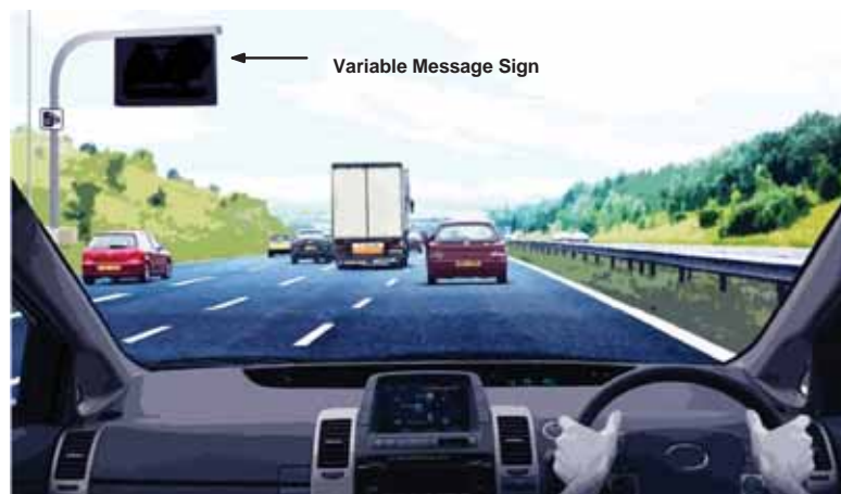
Figure 4B: Illustrative M25MMM section operating in normal motorway conditions with a blank verge mounted Variable Message Sign
