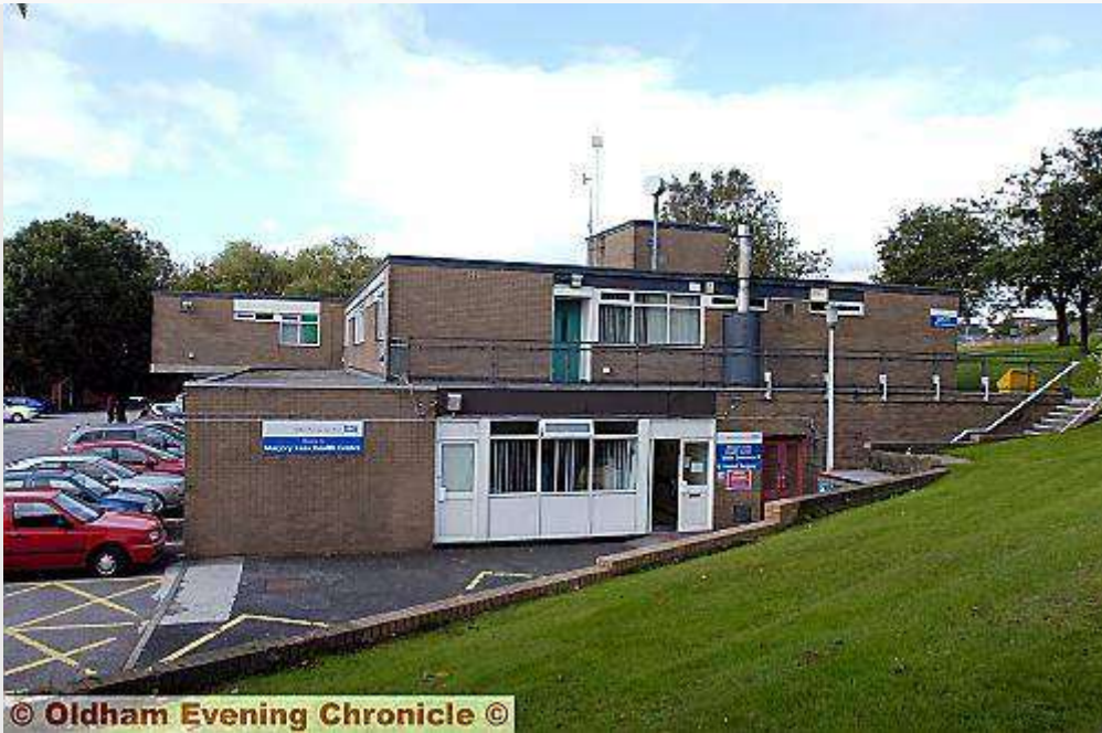
COMING down . . . the Marjory Lees Health Centre will be demolished to make way for the new club © Chronicle Online 17 th September 2009
