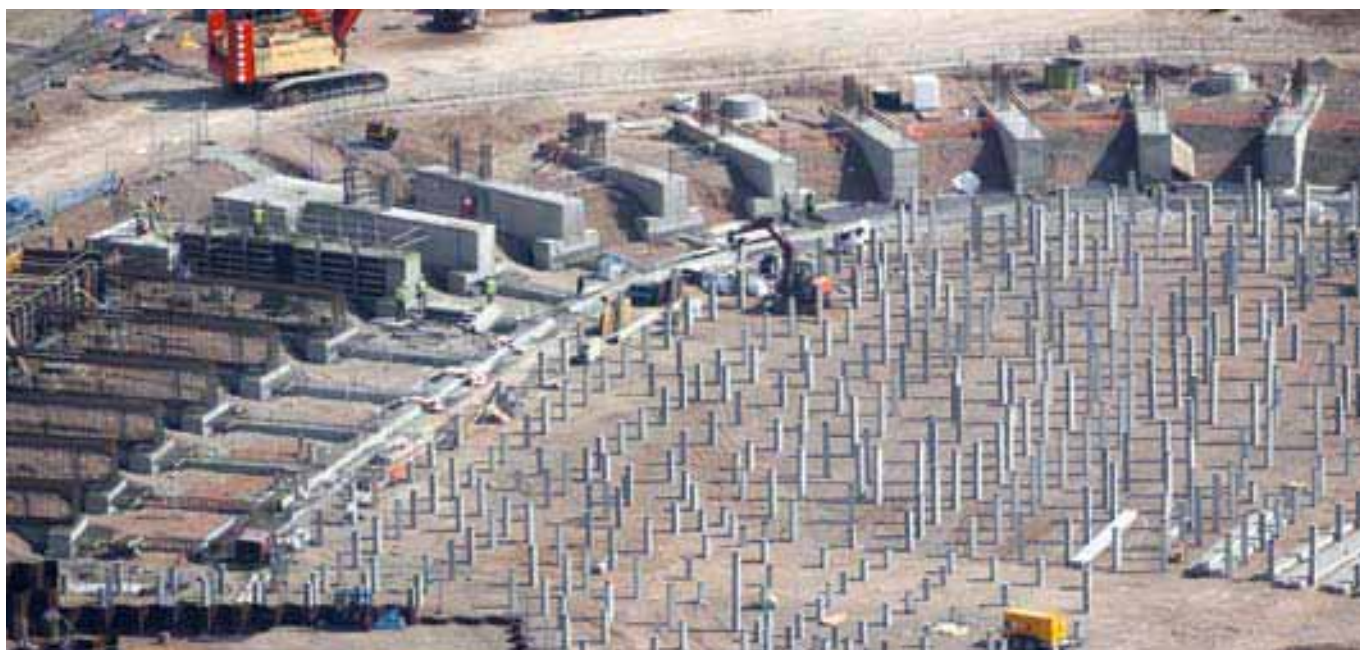
Velodrome under construction April 2009
