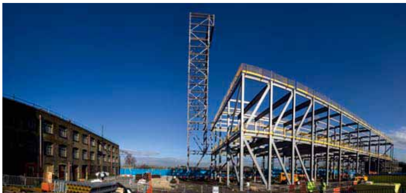
Energy Centre under construction February 2009
