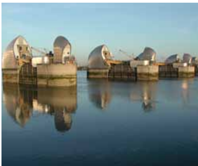
The Thames Barrier (copyright Defra)
