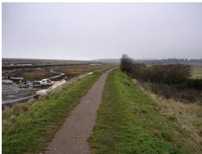
Morston flood embankment
