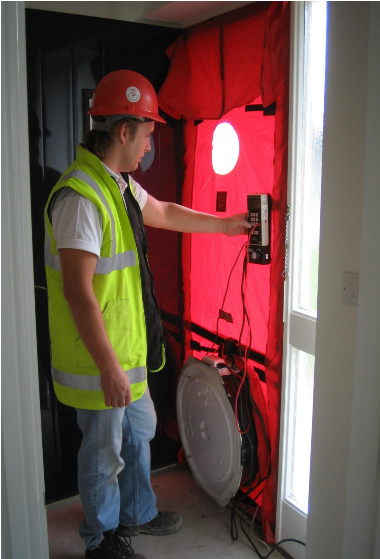
Air tightness testing
