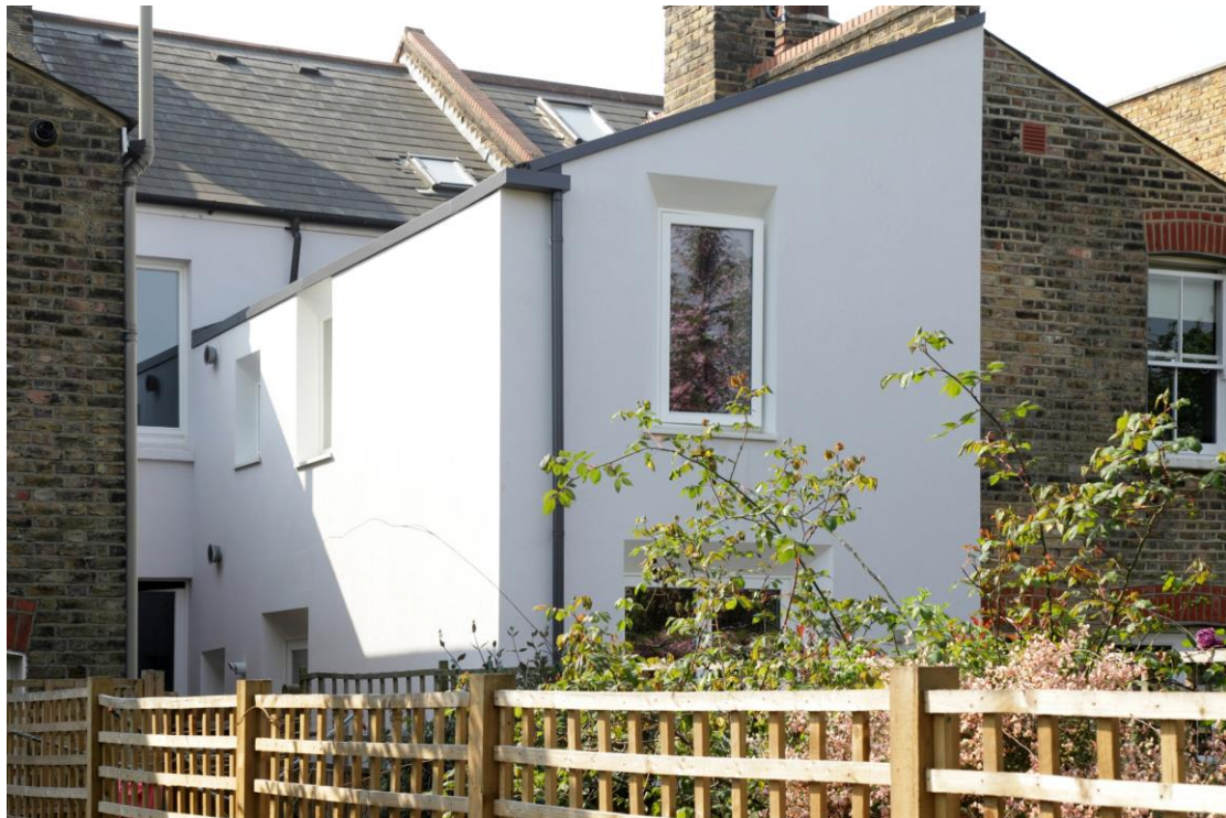
External insulation to a rear elevation
