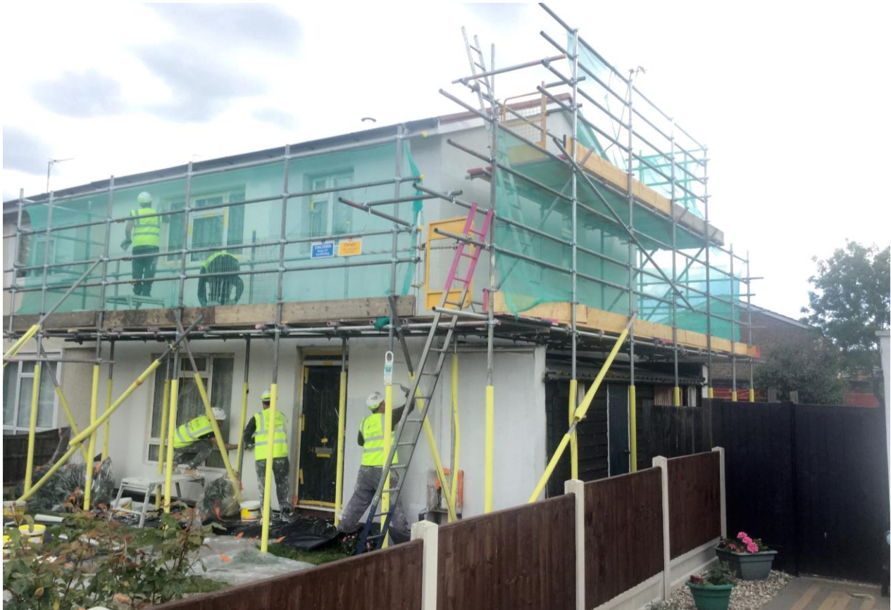
External SWI installation
