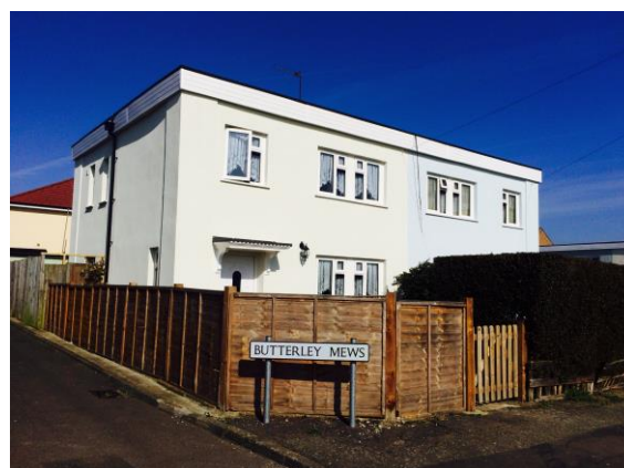
An Orlit type system-built home after external wall and roof insulation
