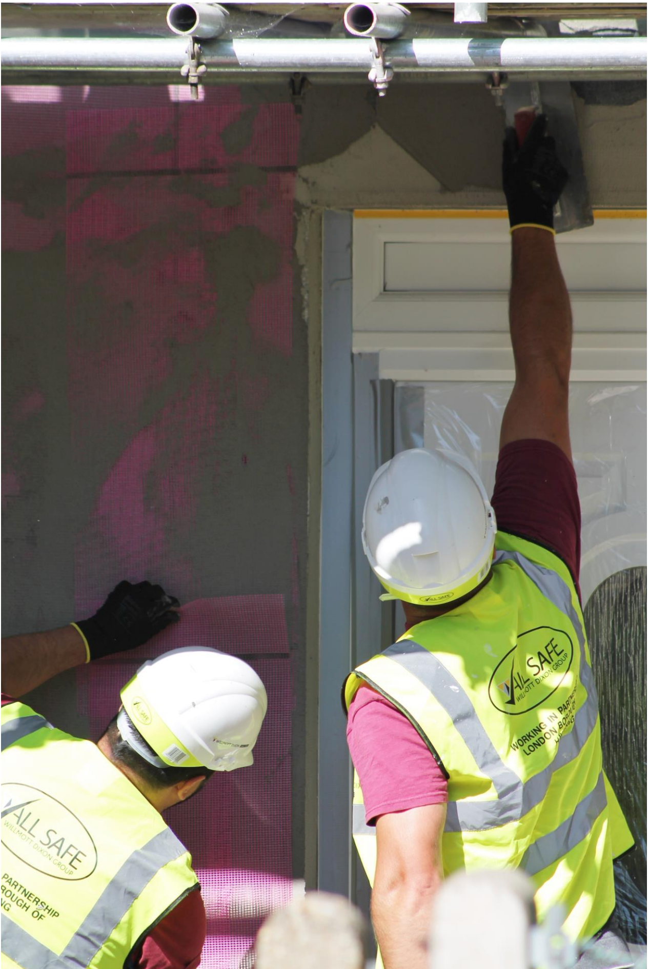
Applying wet trades
