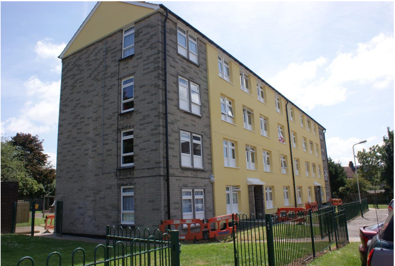
External insulation to social housing block (before and after)
