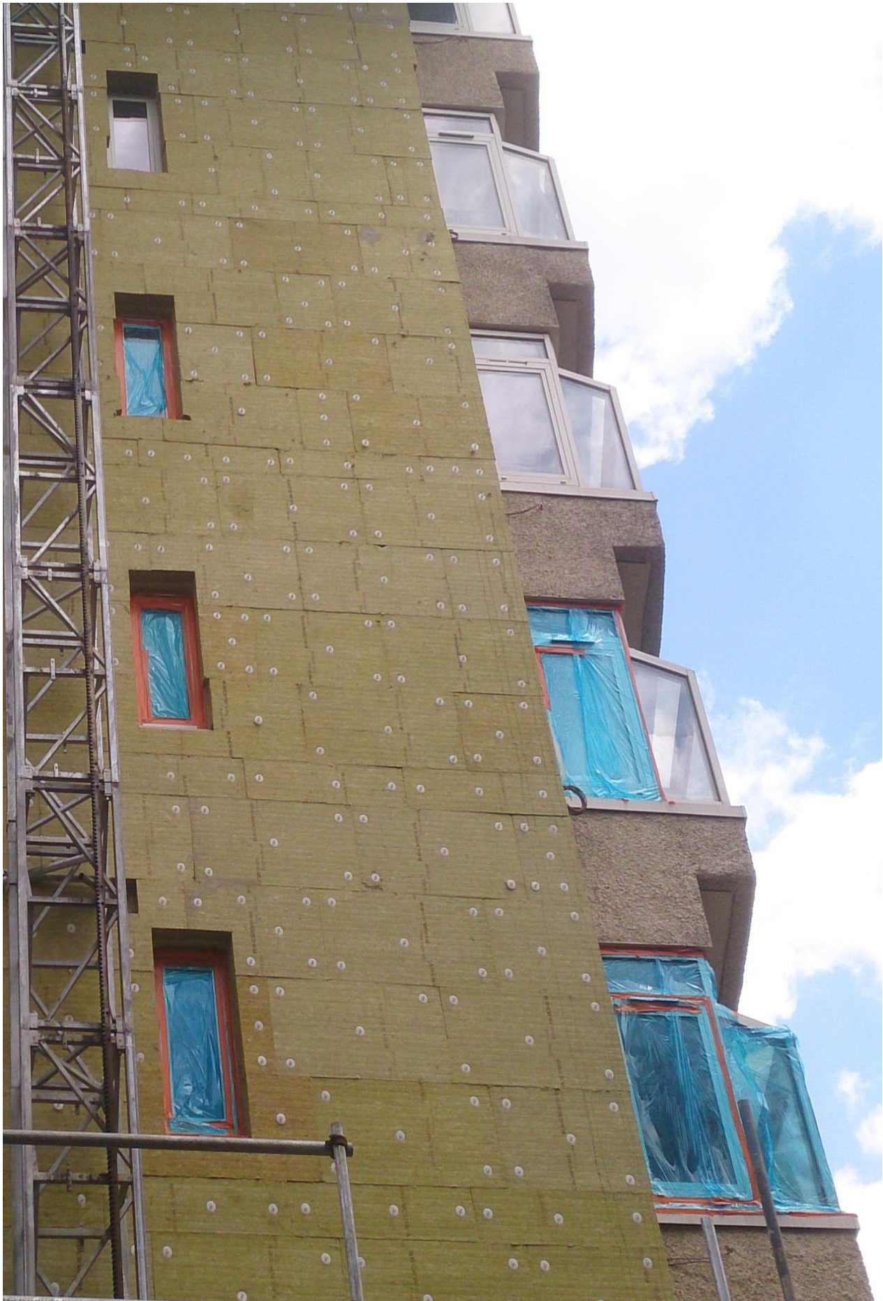
External insulation in progress to high-rise block
