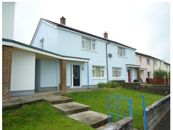
The Beeches, a typical 3-bed semi-detached property after the works
