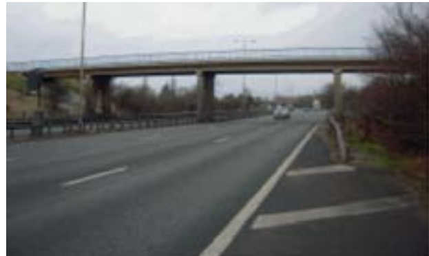
Figure 5: Discontinuous hard shoulder at overbridge
