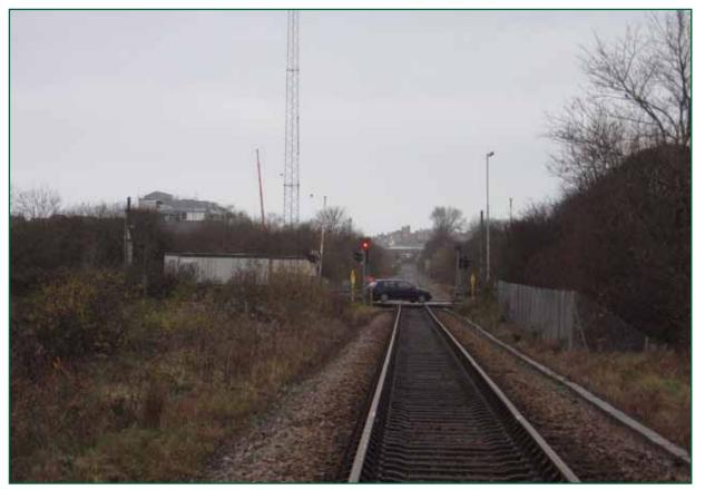
Figure 6: Llanbadarn ABCL showing driver's crossing indicator (flashing red)
