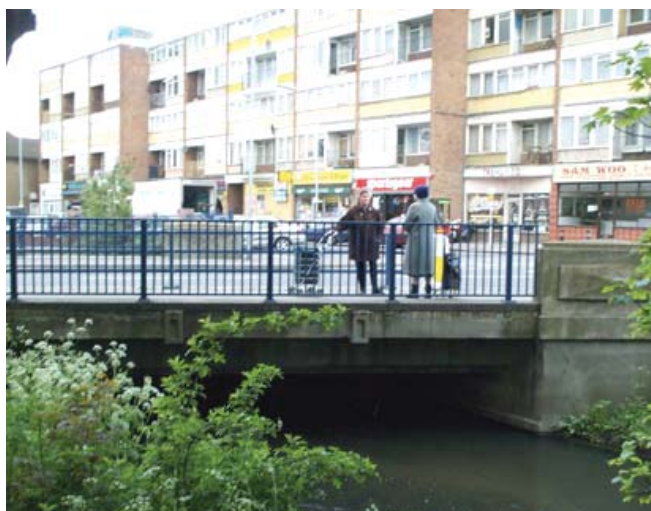
← B2186 Bridge in Crayford.
