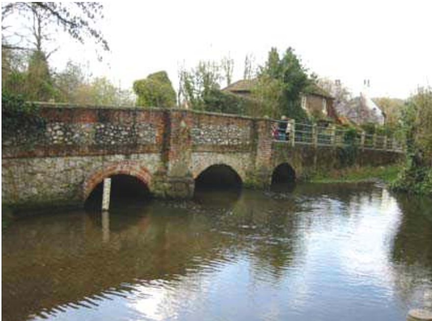
← High flood waters at Church Street Bridge, Shoreham, Kent.
