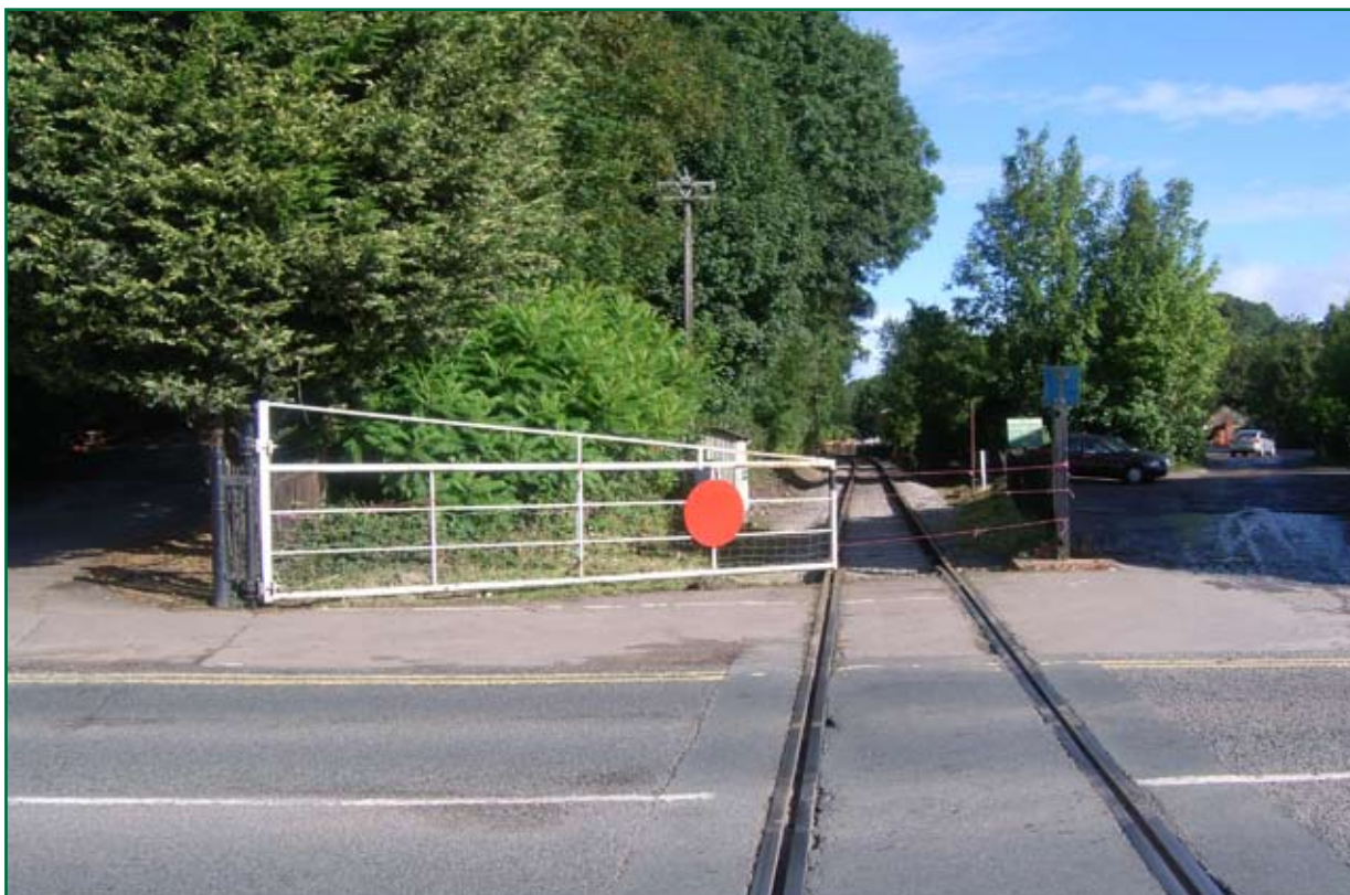
Figure 4: Lydney town crossing looking north (secondary gate missing following accident)
