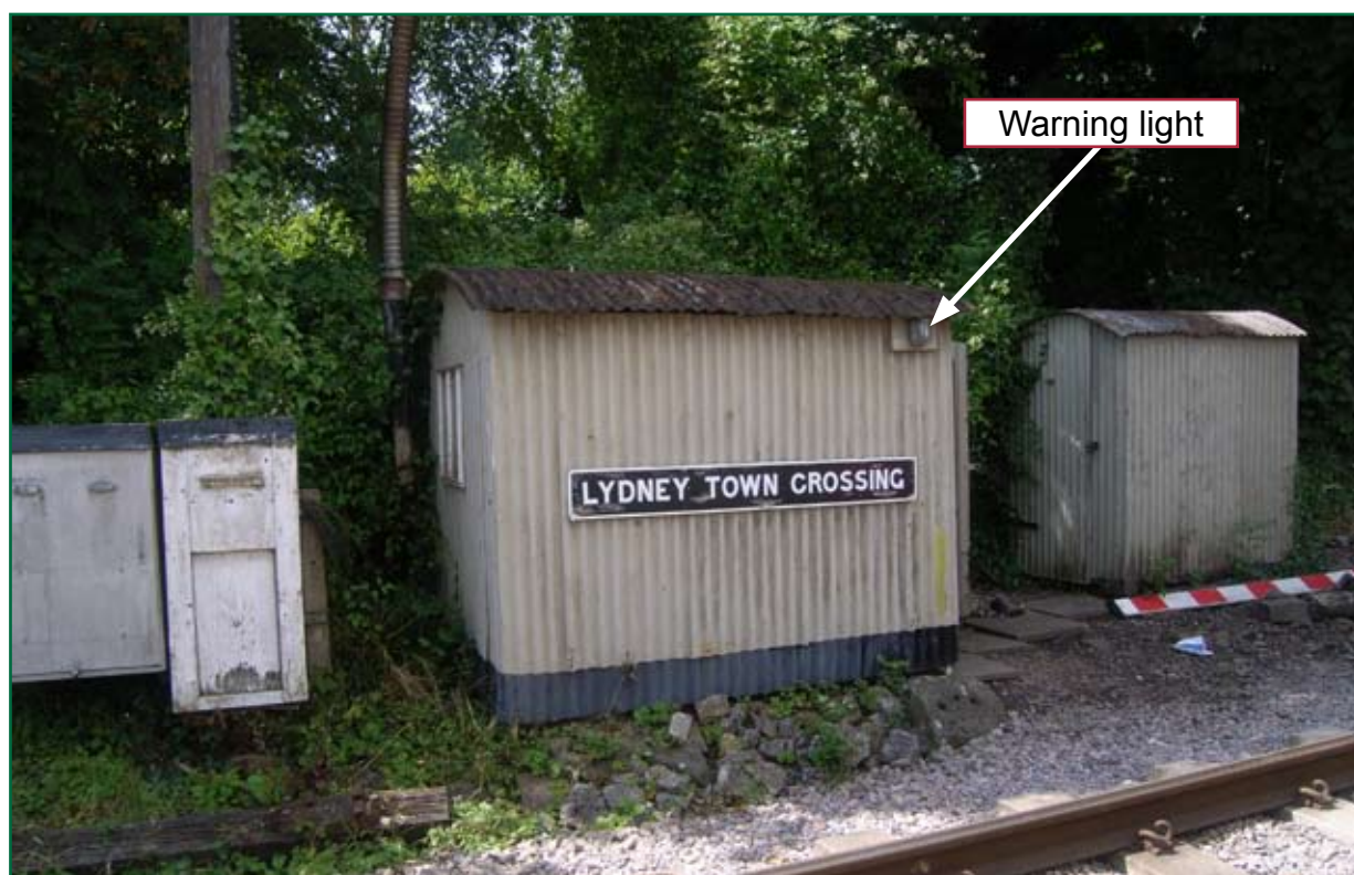
Figure 5: Crossing keeper's hut, showing warning light for approach of trains
