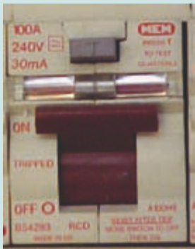
residual current device (RCD)
