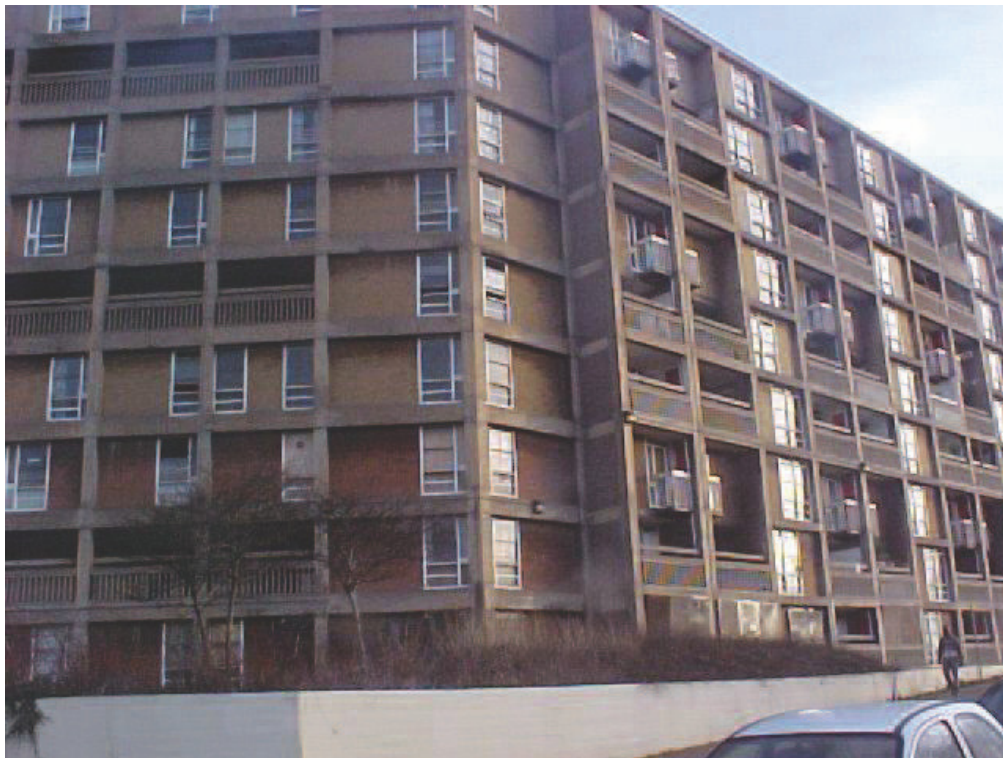
Figure 1.18: A purpose-built block of flats with in-situ concrete frame
