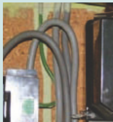
unsheathed or green covered earthing wire
