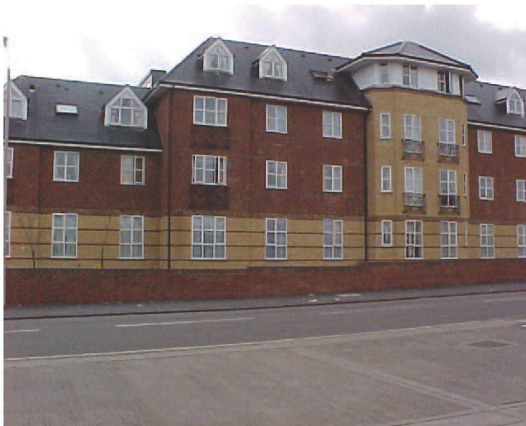
Figure 1.3: Block of flats with rooms built into the roof as part of the original design
