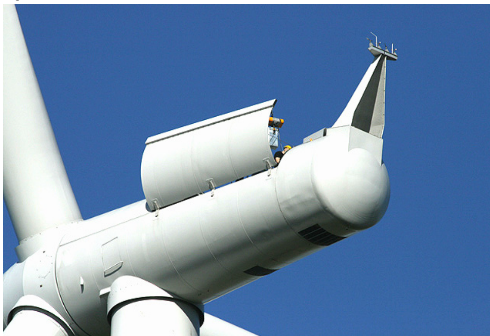
Figure 3-4: Wind Turbine Maintenance at Minsca Wind Farm
