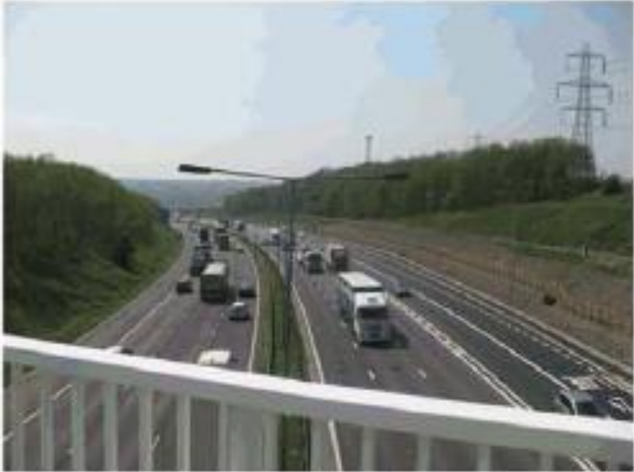
Figure B.1 EnAR Photoview P19 South – before
