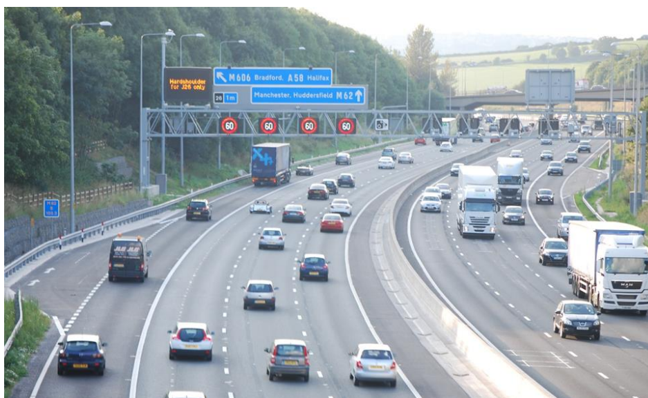
Figure 5-9 Traffic responding to the Gantry signage, using the hard shoulder on the M62 between J27 and 26.
