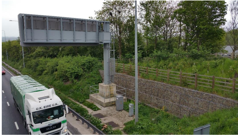
Figure 5-5 Illustration of the successful retention of established vegetation to the upper limits of slopes
