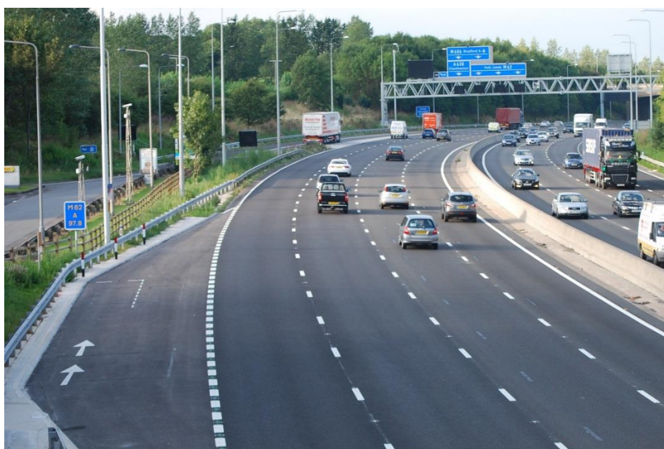
Figure 3-2 Emergency Refuge Area on eastbound carriageway between J25-26
