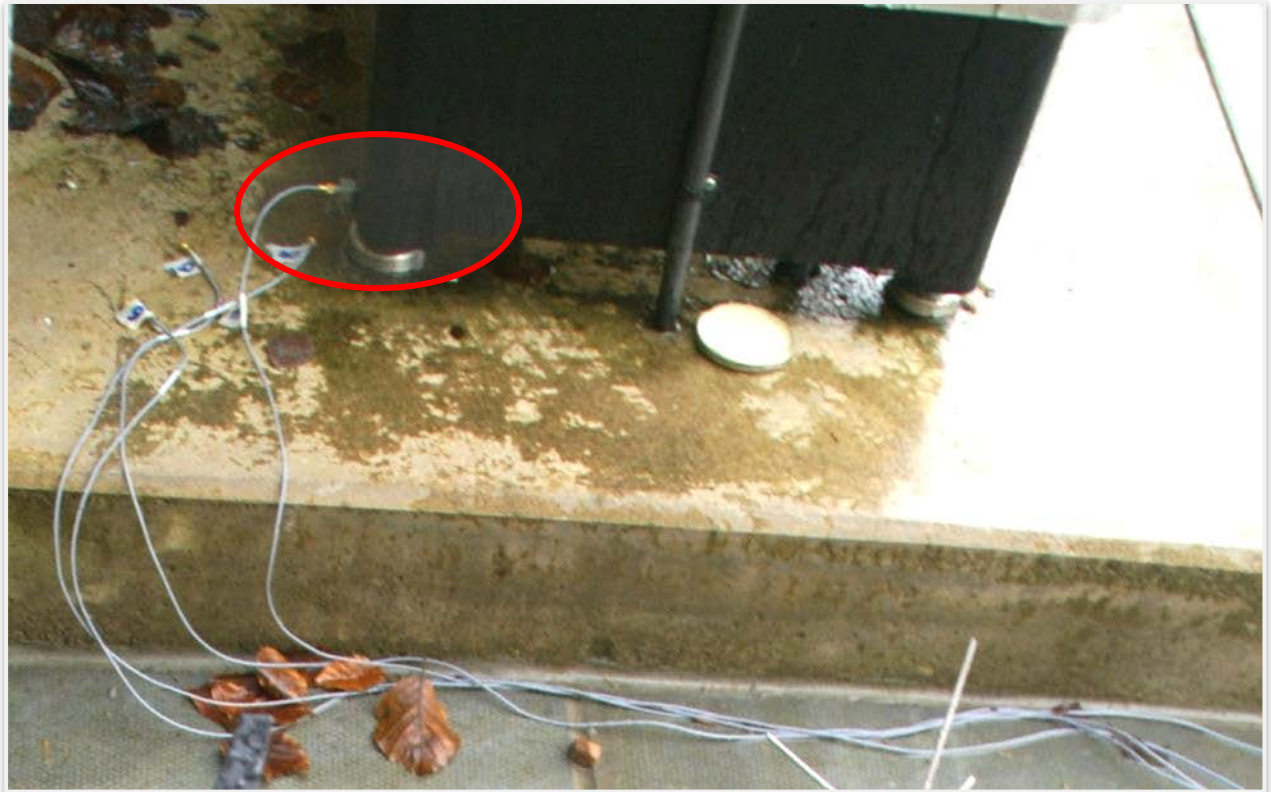
Picture 5-8. 418 Central Buchan, Casing-mounted Accelerometer
