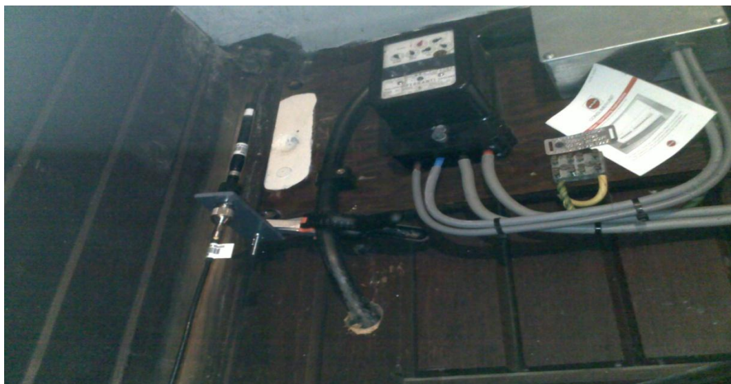
Figure 14: The antenna can be clamped near the Actual meter to match the height of the meter
